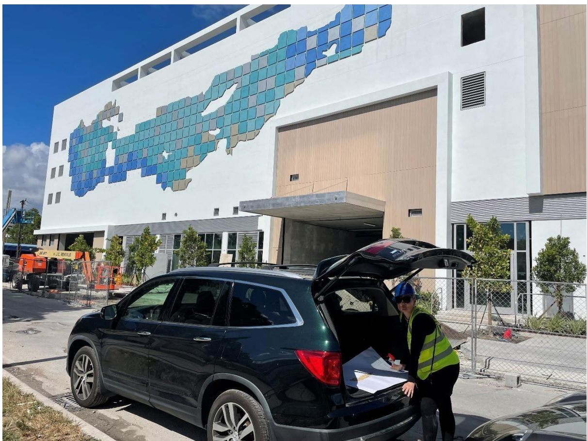
Platform 3750 site visit near completion.
