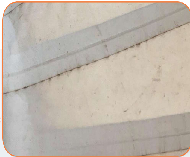
Normal Welding Bump Polyester Fabric Exposed
