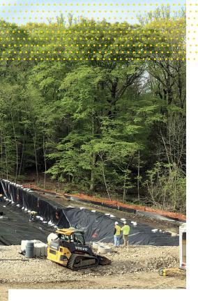
Workers from New England Liner Systems thermal-fusion weld seams where the 40-mil liners overlap in the revetment. (Photos courtesy of Green Construction Management)
