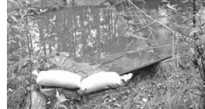
Above: A number of silt fences and silt trap pools were in place along the stream channel, during the restoration program. This was carried out to reduce the amount of silt loading into the Bigbill Creek and Bow River, downstream. These pools and fences were maintained daily.
