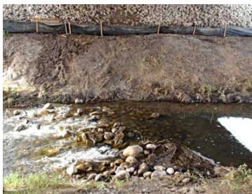
Above: Bow Valley Habitat Development volunteers modified this rock dam that had been constructed by kids, underneath an overpass, using rock that was intended to armour the bridge. The modifications allowed brown trout to migrate up the stream to spawn this year. The modifications only took minutes to complete, yet the result produced a total of 11 trout redds further upstream. Not a bad return for a few minutes of work.
