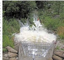
These photos show a typical length of channel on Ranch House Spring Creek, prior to the installation of the storm drain, in to the creek channel.
