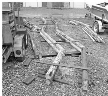
Above: The log retaining walls for the spawning channel were constructed off site and then transported to the spring channel for installation.
