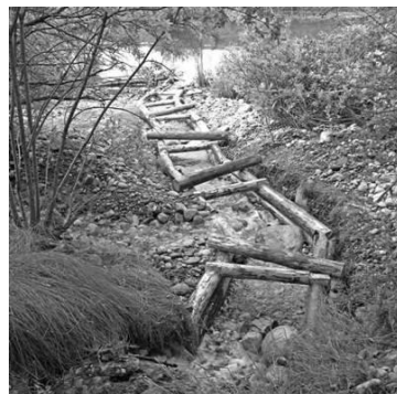
Above: This photo shows how the channel looked, just after it was installed in the excavated spring channel. The log retainers kept the channel's loose gravel in place.
