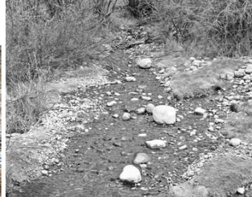
Above: This is what the spawning channel site looked like, before the excavation took place. There was plenty of good spawning gravel, but not adequate flow and depth. Much of the main volume of flow was subsurface. By excavating down and concentrating the flow into a narrow channel, the site would be transformed into a spawning channel.
