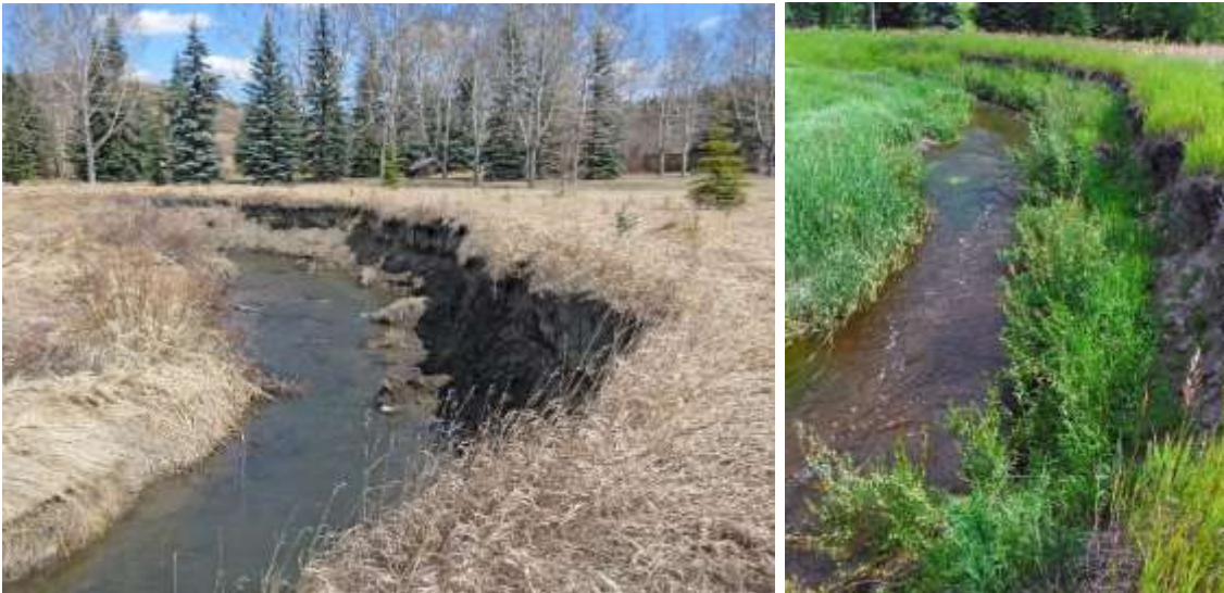
Above: This eroding stream bank stabilization project was completed entirely by using Stage One, push plantings in the applications. The photos are five years apart.
