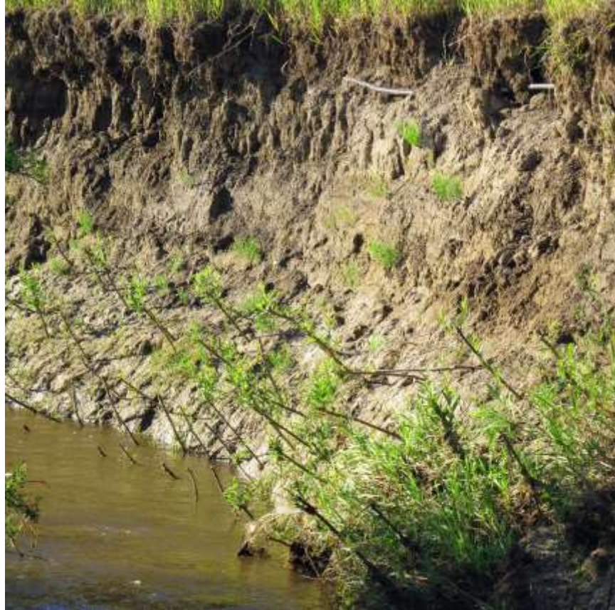
Above: An eroding stream bank that has just been planted. Check out the follow-up photo below. You will see quite a dramatic result after only a few years of growth.
