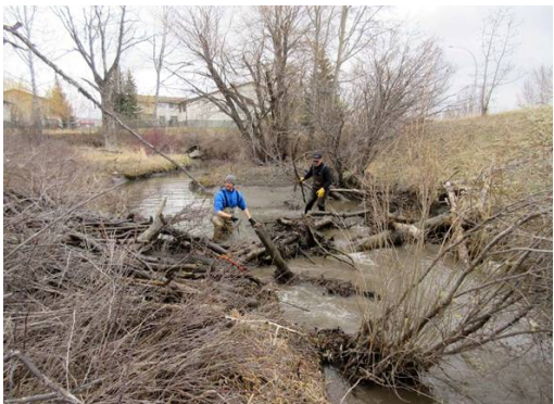
Above: The mature willow in the centre of the stream channel in this photo is still alive, so dead woody debris was removed from a blockage that the tree had created, allowing trout migration up past the old willow's location.
