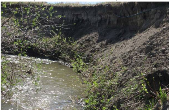
Above: Eroding stream banks like the one pictured above are responsible for loading tonnes of silt annually into the stream channel on the Bighill Creek. By planting Stage One willow cuttings in the most area at the base of the steep slopes, the erosion impacts will start to reduce and eventually the steep banks will stabilize over time. This is the most cost effective method of dealing with problem sites such as this one. The banks require a number of treatments (plantings), in the first attempts to establish willow plants, but it is still worth the effort.
