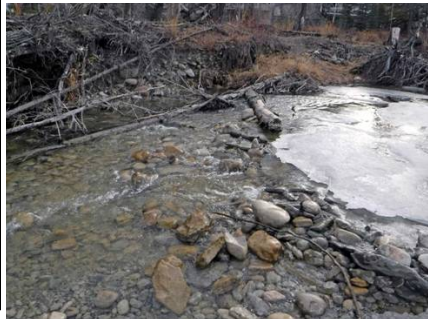
Below: This is what the dam looked like, after the middle of the dam was opened up. The water level in the creek at the time of the notching of the dam, was very low seasonal flow.
