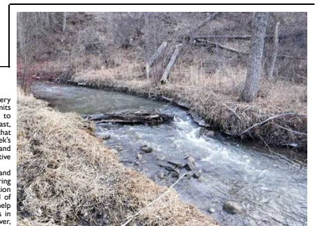
Above: This blockage was causing the stream's flow to start eroding into the far stream bank. It also constricted the flow for trout migrating up the system.
