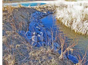
Above: Rip-Rap rock is commonly used for stabilizing eroding stream banks. The ruff quarry rock is placed on the outside banks of stream channels to prevent toe erosion. This measure greatly reduces the amount of silt loading into the stream channel and this will improve the water quality in the stream and help keep the streambed free from a thick layer of silt. The size of rock used is dependent on the mean average volume of flow in the stream and how high the spring run-off is.
