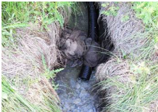
Above: A flow-by-pass pipe was used to isolate the work area on the stream channel. This would insure no silt loading into the creek.
