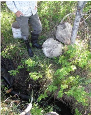
Below: Large rocks were installed on opposing sides of the stream channel, to create a stepping down of the steep gradient. This would allow easy migration of trout into the middle and upper reaches of the stream. There had been no trout found upstream of the waterfall.
