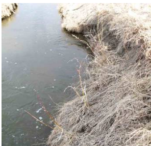
Above: This photo shows one of the stream bank stabilization sites on West Nose Creek, which have been planted in previous years. You can see the new willow growing on the unstable soil of this eroding stream bank. This site is one of 96 stabilization sites that have been planted on the West Nose Creek, in the city.
