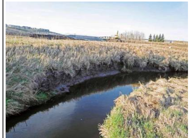
Above: This eroding stream bank on West Nose Creek is actively in a state of collapse. Water eroding the base or toe of the outside stream bank is causing the stream bank failure.
