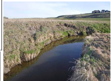
Above: This is another example of an eroding stream bank on West Nose Creek.
