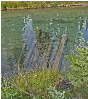
Above: This is a photo of one of the deflectors that Bow Valley Habitat Development installed on Polkeman Creek, in the Town of Canmore, Alberta. The project had been completed a few years before this photo was taken.
