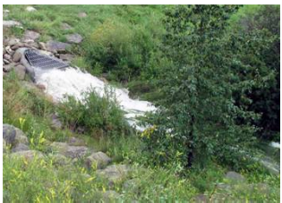
The outflow of a storm drain on RHS Creek, during a rain event in the residential development. The development is located just on top of the Bighill Creek Valley. This was from the Phase One development, now there is a Phase Two tied into the same outflow.
