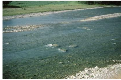
Above: This is what one of the triple rock placements looked like in 1996, just after the project for that year was completed. Note the pocket pool area just below the three rocks. This provides great low water fish habitat!
