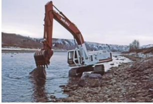
Above: In 1987, a series of very large boulder rock placements were completed on the Bow River in the Town of Cochrane. The objective was to create low flow habitat for trout and mountain whitefish.
