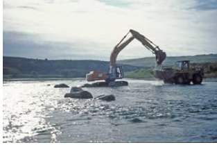
Above: In 1996, a much larger boulder fish habitat enhancement project was completed at five different sites on the Bow River in the Town of Cochrane, Alberta. In total, a 133 class 4 and 5 boulders were placed in the riverbed at sites.
