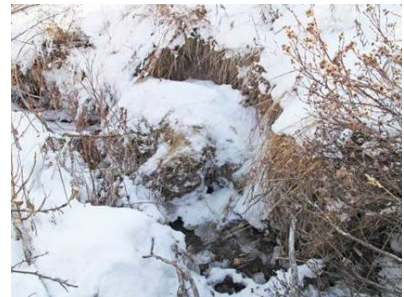
Above: This January 2012 photo shows the collapsed stream bank that occurred in 2011 on Ranch House Spring Creek, approximately 60 metres downstream of the storm drain outflow.
