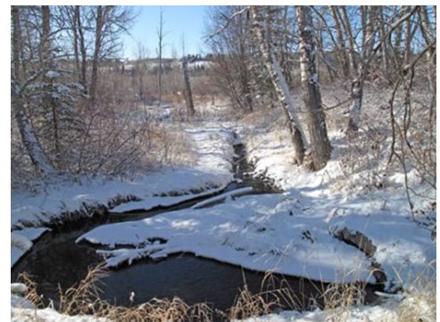
Above: This February 2012 photo shows the new stream channel that was cut thru this section of the stream in 2005. Now there is a defined narrow channel that supports a resident trout population. Over time, the willows that were planted along the channel downstream, will hide much of this reach of stream channel, but the plants will help maintain stability in the stream banks!
