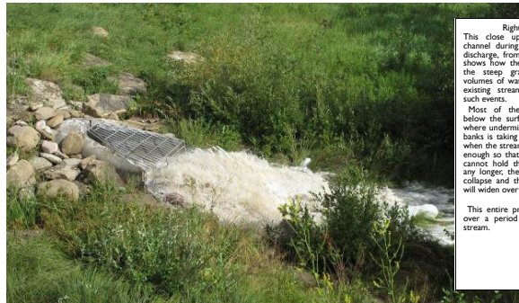
Above: This photo shows the volume of flow added by the storm drain from Sun Ridge in August of 2010. This volume of flow is approximately 10 times what the natural channel can handle.
