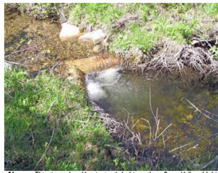
Above: This is a log V-weir pool habitat that Bow Valley Habitat Development designed and constructed. The photo was taken four years after construction was completed. The structure is starting to blend in.
