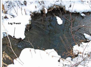
Above: You can see in this photo that the log v-weir has a very minimal hydraulic jump, yet it maintains a deep pool habitat with lots of cover for resident trout.
