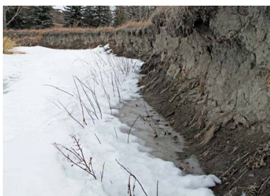
Above: This is one of 58 stream bank stabilization sites on the Bighill Creek, which is part of the "Bow Valley Riparian Recovery and Enhancement Program". It has taken a few years to get this far, but the results are now evident for future success. The native willow plants stand out in the winter snow covered ice of the Bighill Creek. (See Page 4)
