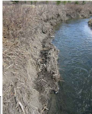
Above: Before photo, this eroding stream bank on Biggill Creek was planted with native willows to help stabilize the eroding bank.
