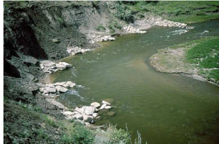
Above: This is a 1997 photo of the site, one year after completion.
