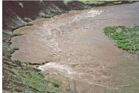
Above: This is a photo of the site during the spring run-off event in 1997. Note: You can see how the deflectors keep the fast flow velocity away from the base of the steep bank to the left side of the channel.
