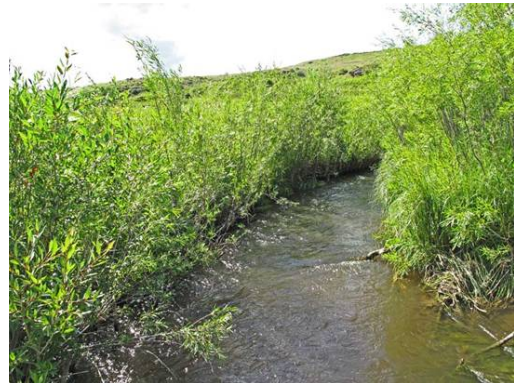
Above: This is a 2011 photo of the wattle fence (left side of the stream channel) that was constructed along the outside bank of a meander on Bighill Creek, in 2008. The project was completed by volunteers from the Branches and Banks Organization, based out of Cochrane, Alberta.
