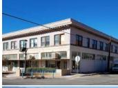
**BISBEE**: The Cole Building is located in the Warren neighborhood and was built in 1909-1910. Formerly known as the McGregor Building and the Warren Hotel, it is made of steam cured concrete block with a fixed steel storefront.
