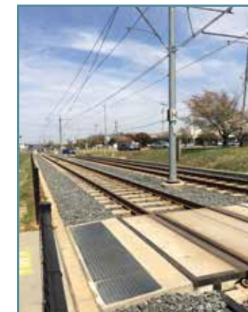
Figure 6: Charlotte LYNX System - Ballast Curb
