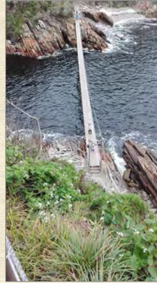
Storm's River suspension bridge
