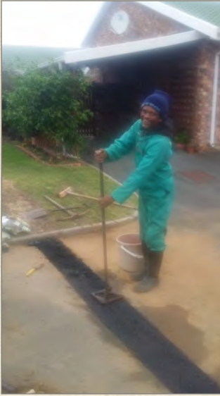
Workers in our compound doing some asphalt work.
