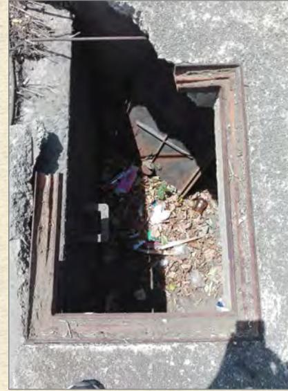
Another manhole type covering that is missing (actually fallen into the hole). We need to get it fixed before there is a serious accident.
