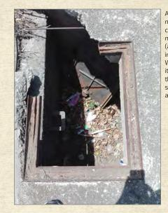
Another manhole type covering that is missing (actually fallen into the hole). We need to get it fix before there is a serious accident.
