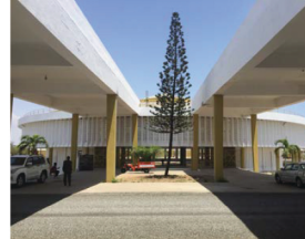
ROUND PAVILION, 2018 VICTOR ADEGBITE, MASTER PLAN; DESIGN BY JACEK CHYROSZ & STANISLAW RYMASZEWSKI
