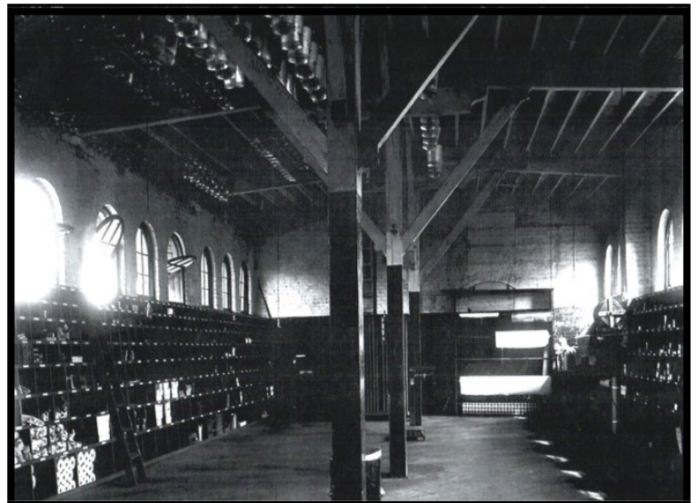
Historic 1915 photograph of Storehouse interior
