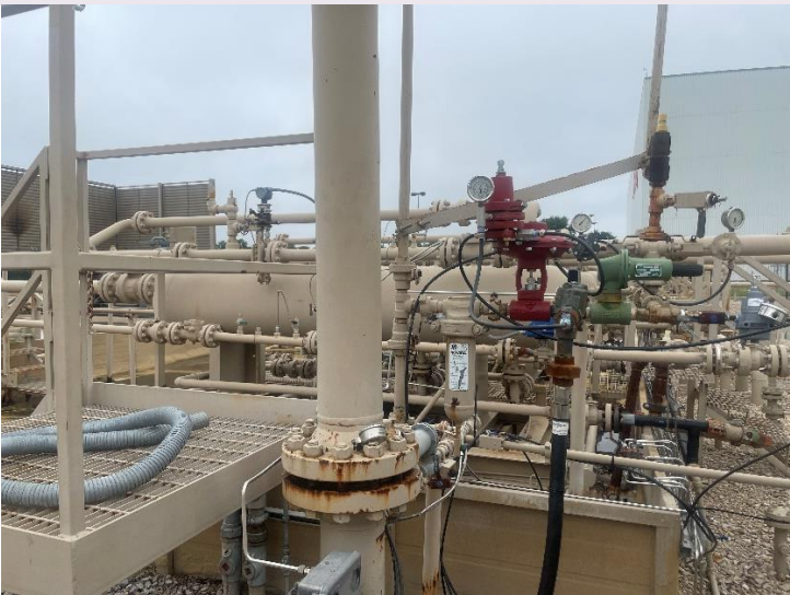
Figure 10: . . . for compressed air pneumatic valve (painted red)
