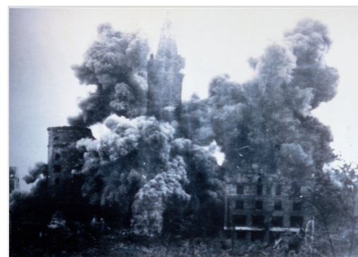
Demolition of the Königsberg Castle with explosives, 1959
