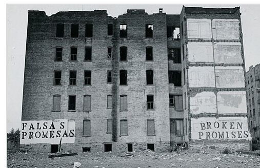
Urban decay in the US: the South Bronx, New York City, was exemplar of the federal and local government's abandonment of the cities in the 1970s and 1980s; the Spanish sign reads "FALSAS PROMESAS", the English sign reads "BROKEN PROMISES".
