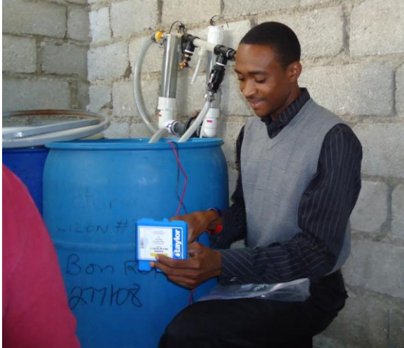
Josue' installing a new water system.
