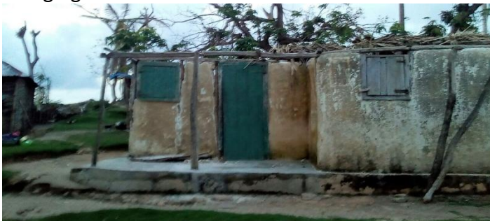
Roof blew off during the hurricane. We sent food and clothes and helped replace a roof.
