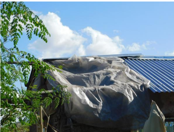
Roof needing repairs
