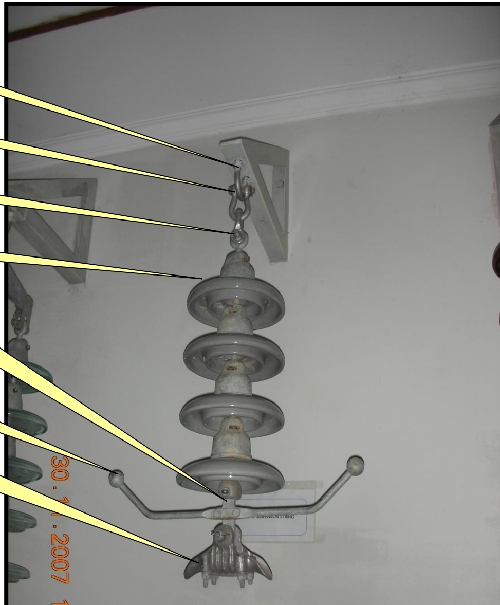
Suspension Insulator String
