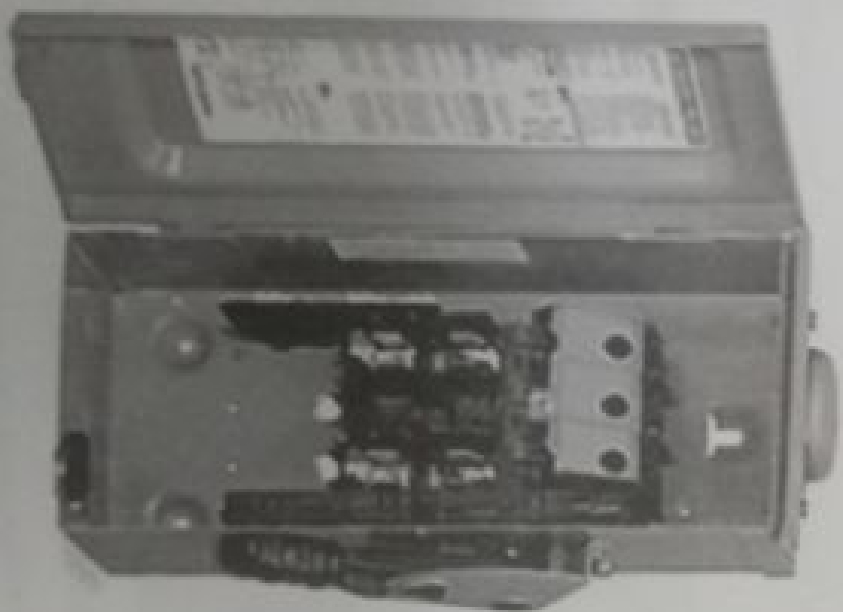
AC Disconnect Switch
