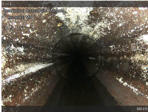
Access Point Manhole at 000.0 ft | MH 1
