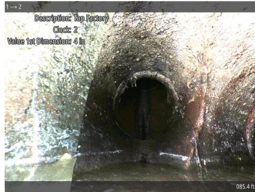
Tap Factory at 085.4 ft, 2 o'clock
