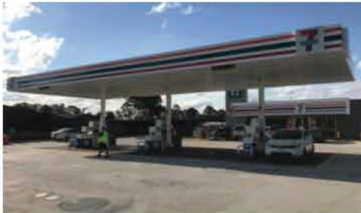
Great Western Highway Werrington NSW
