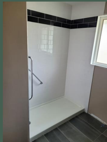
The new walk in shower
