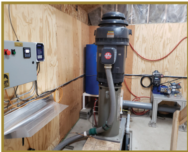
Snow making system and Horner controller panel
