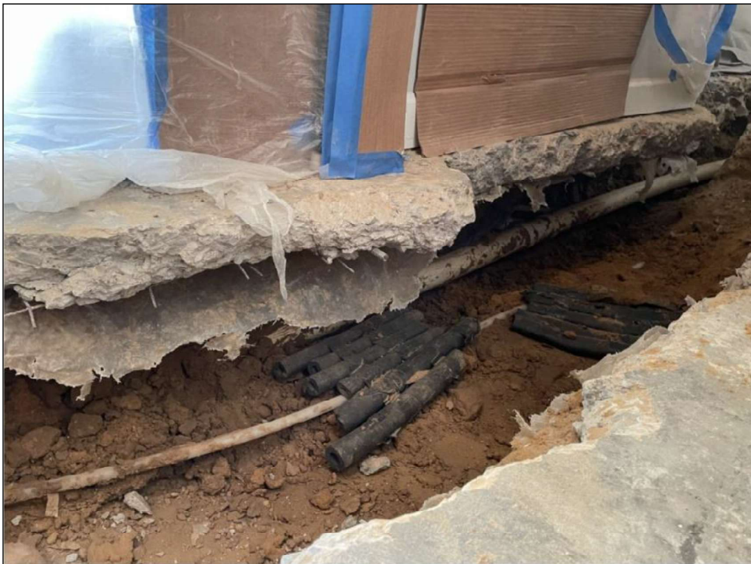
Figure 3 —Photograph taken by homeowner during plumbing repairs, which required partial demolition of main slab. The Welded Wire Reinforcement (WWR) is observed to be lying directly on top of vapor retarder.
