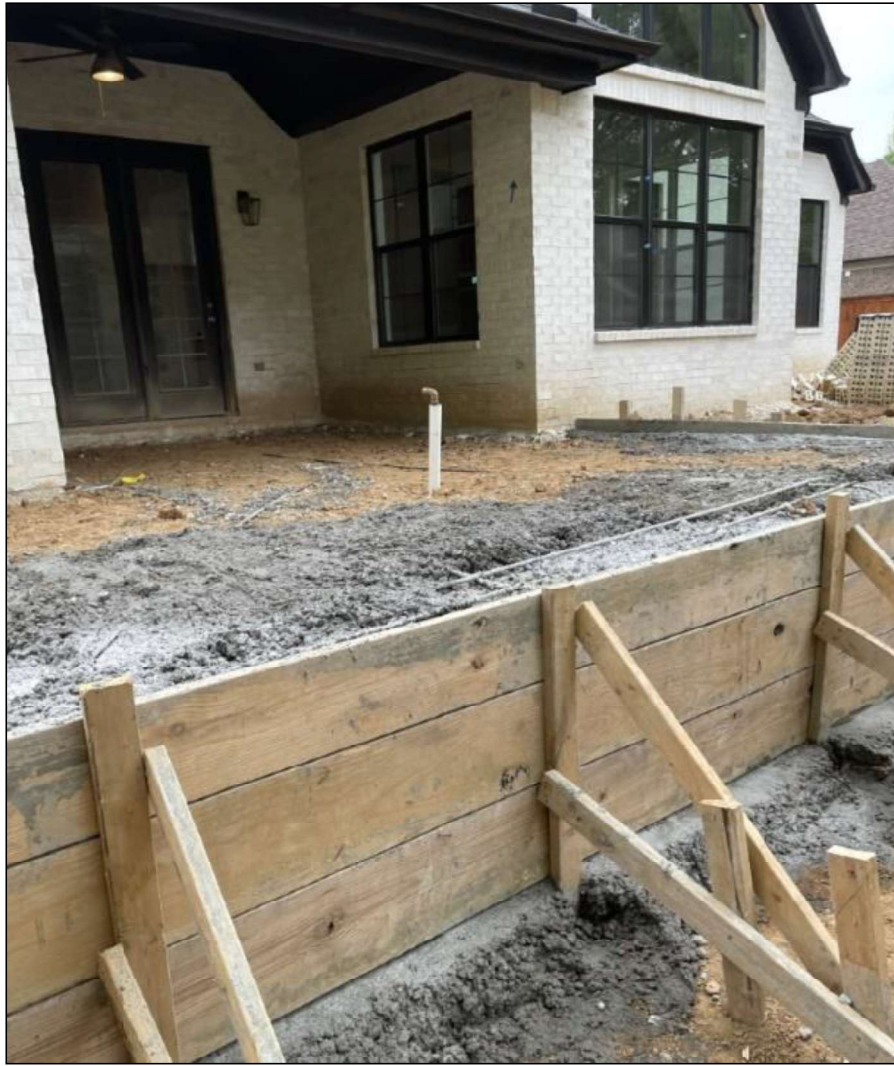
Figure 4 —Photograph taken by homeowner during placement of OLA patio slab. Steel reinforcement is observed to be lying on the ground.
