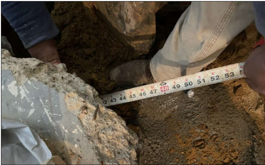
Figure 2 - Photograph taken by homeowner during plumbing repairs, which required demolition of main slab. Tape measure is inserted in area of required 30-inch by 30-inch footing.
