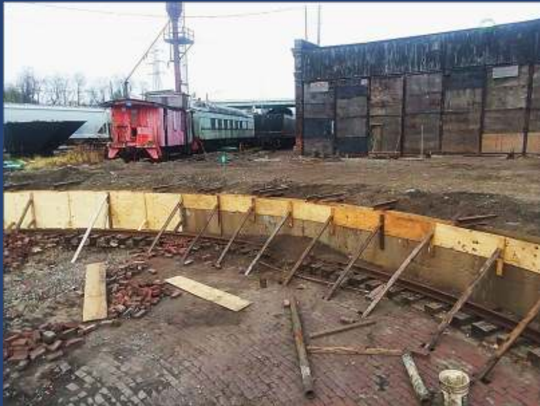
Repairing Turntable + Expanding Tracks
