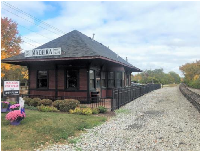
Madeira Station “Before”
