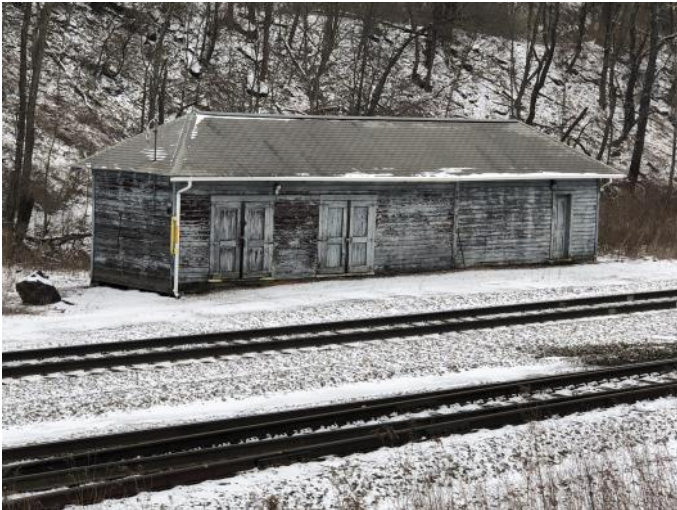
Close up of Section House
