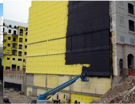
Air Barrier Application
