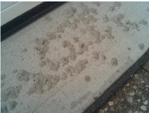
*As you can see this is pitted/spalled and if the MG-Krete overcoating performed like this, debonding internally within MG-Krete 1260, Imco Technologies will supply the repair material but not labor. This debonding/delamination is defined as the MG-Krete leaving the substrate with less than 30% of the substrate attached. If the substrate in excess of 30% is attached this is not a failure of MG-Krete.*
