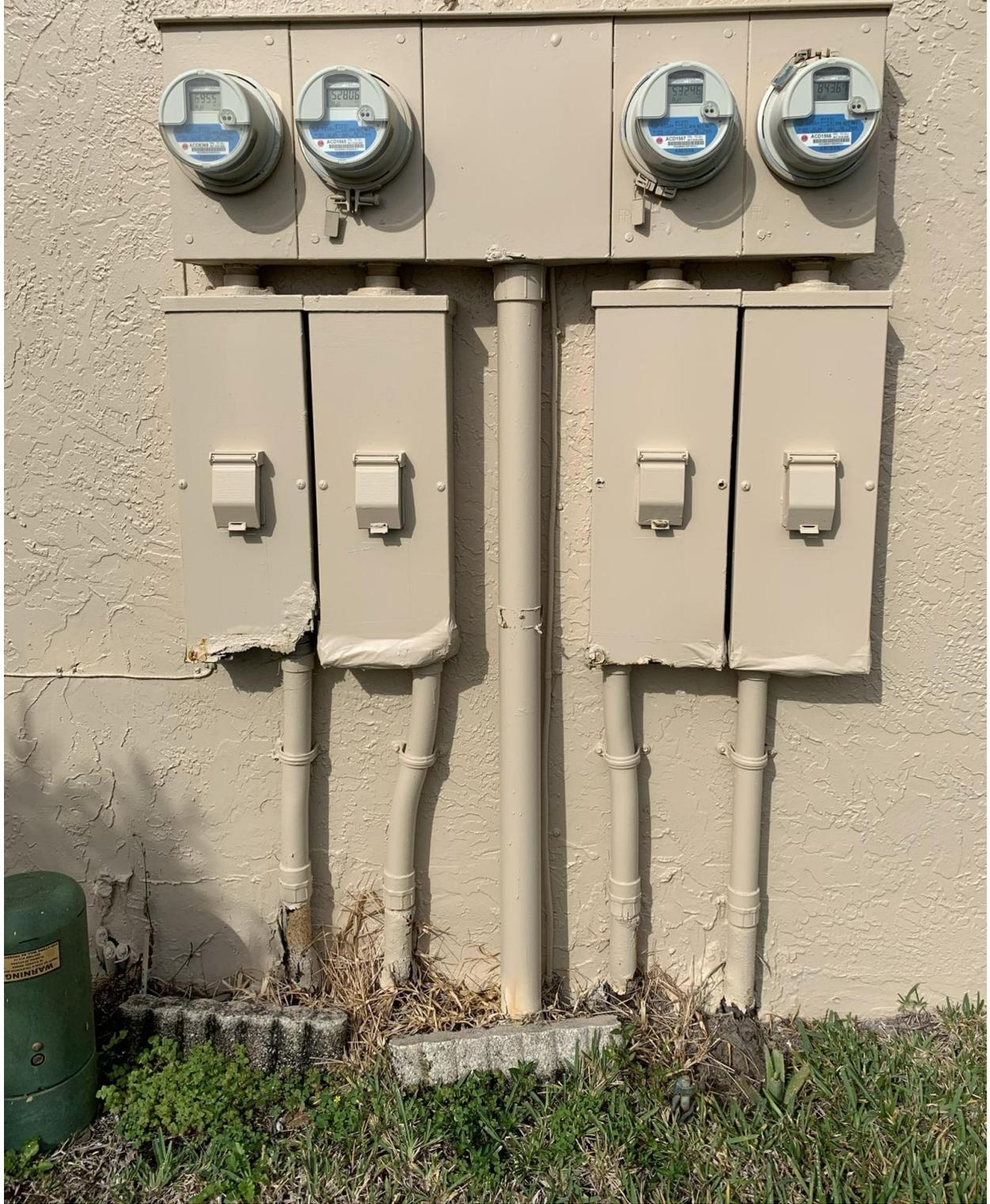
Units 33-36 seem mostly OK; corrosion on bottom of 2<sup>nd</sup> conduit. Replace in 2021.
