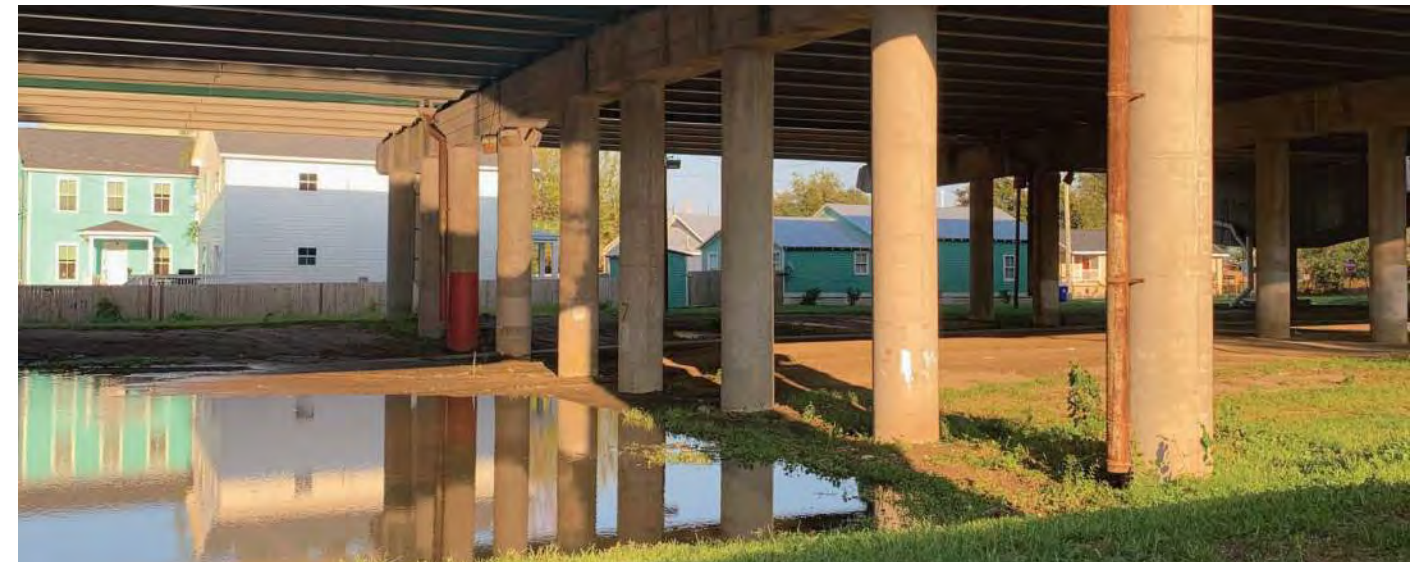
Current Site Conditions: Stormwater from Hurricane Dorian
