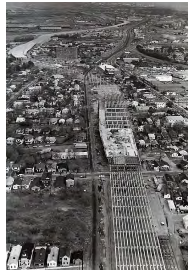
Image of I-26 being constructed 5
