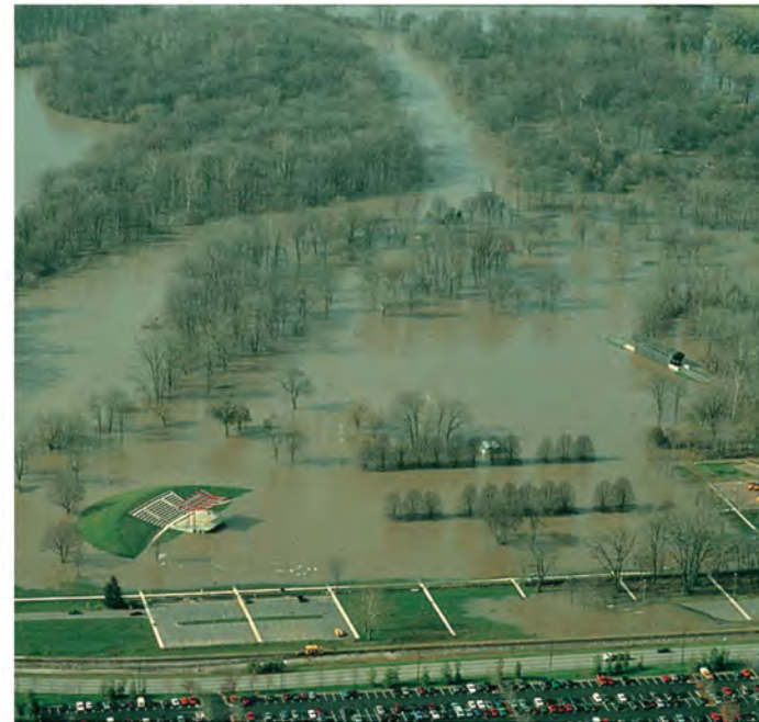
The park is designed to accommodate seasonal flooding from two rivers.
