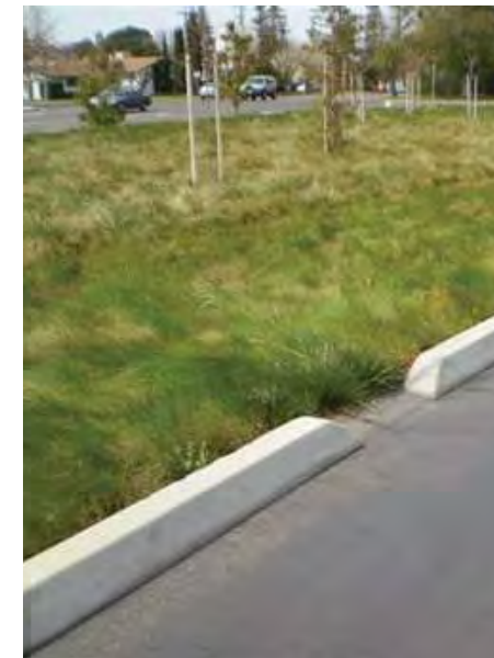
Curb cuts to rain gardens
