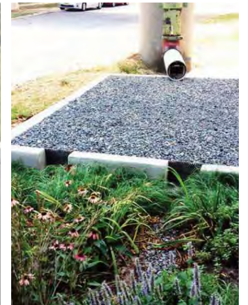
Retrofitted downspout
