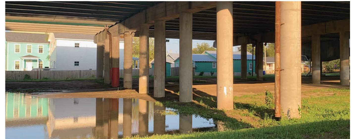
Site Conditions: Stormwater from Hurricane Dorian
