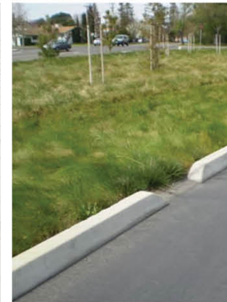
Curb cuts to rain gardens
