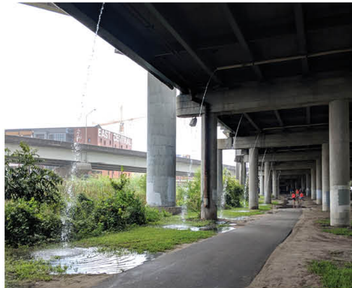
Site Conditions: Runoff from the overpass
