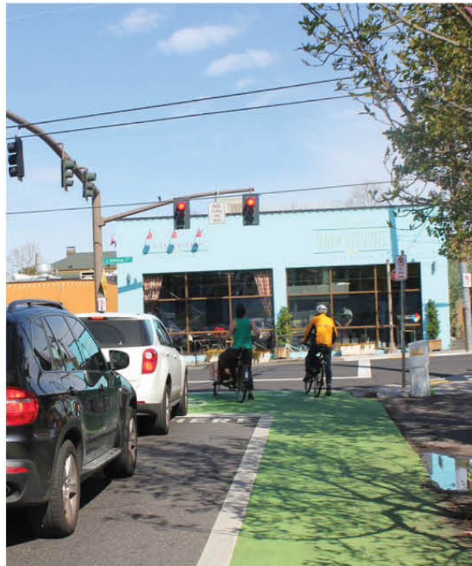
Example of a painted bike lane with a bike box at the intersection.
