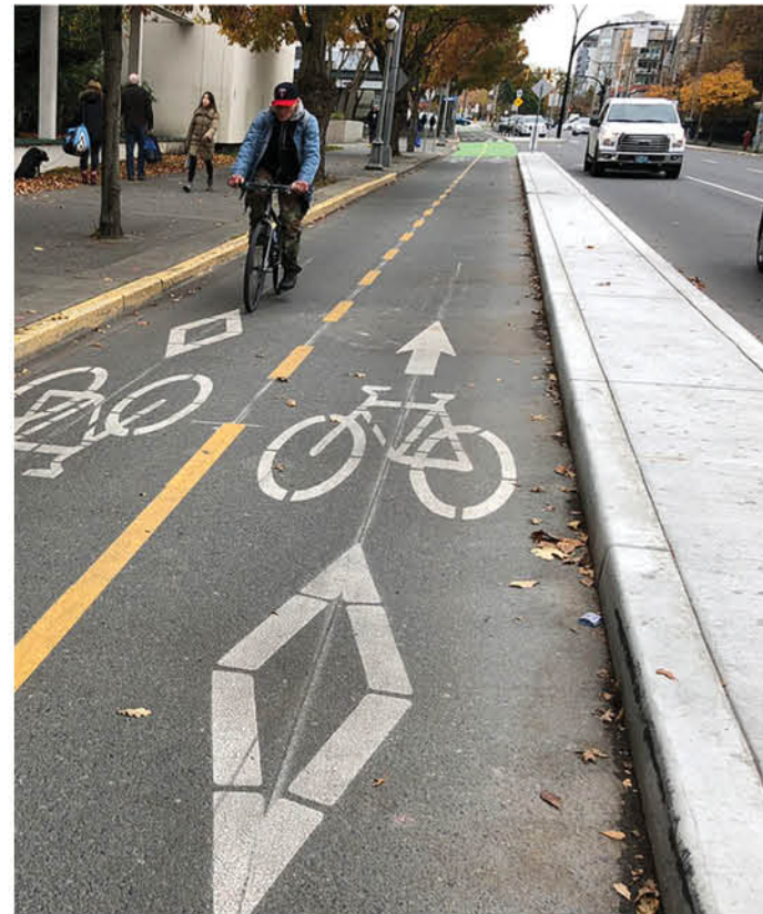
Example of a separated two-way cycle track.
