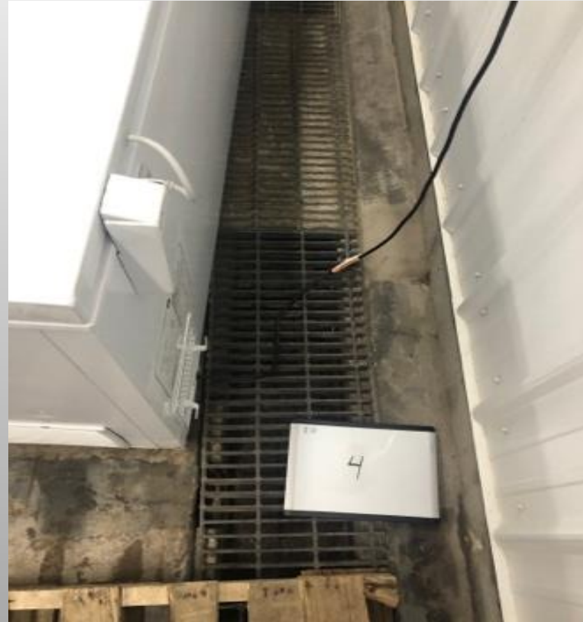
Truck bay drain (CO4)
