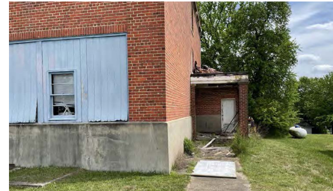
Source: Stantec - Photographic log
