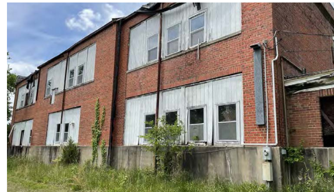
Source: Stantec - Photographic log
