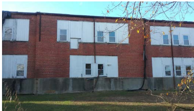
Source: Stantec - Photographic log
