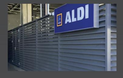
Two Point Seven Facades Ltd provided the full turn-key package. We performed the design, manufacture and installation of aluminium louvres to plantroom ventilation.
