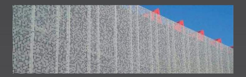
Perforated cladding provides a practical purpose, too. Depending on the size of perforations, the amount of natural light reaching the inside of the building can be managed. Large perforations allow more natural light to pass through the cladding, but still protect buildings that have large glazed elements from direct sunlight. In doing this they reduce the amount of solar gain, mitigating the need for energy intensive air conditioning systems.
