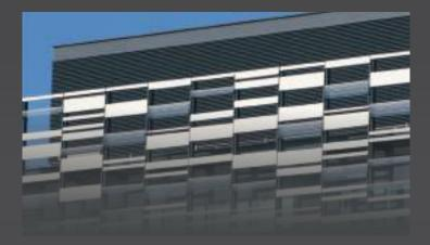
Cantilevered sunshades are ideal for both new and existing construction. They provide effective shading while maintaining unobstructed views. Projection and blade size may be varied to suit the project requirement.
